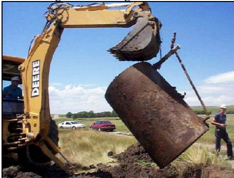
Underground Storage Tank Removal
